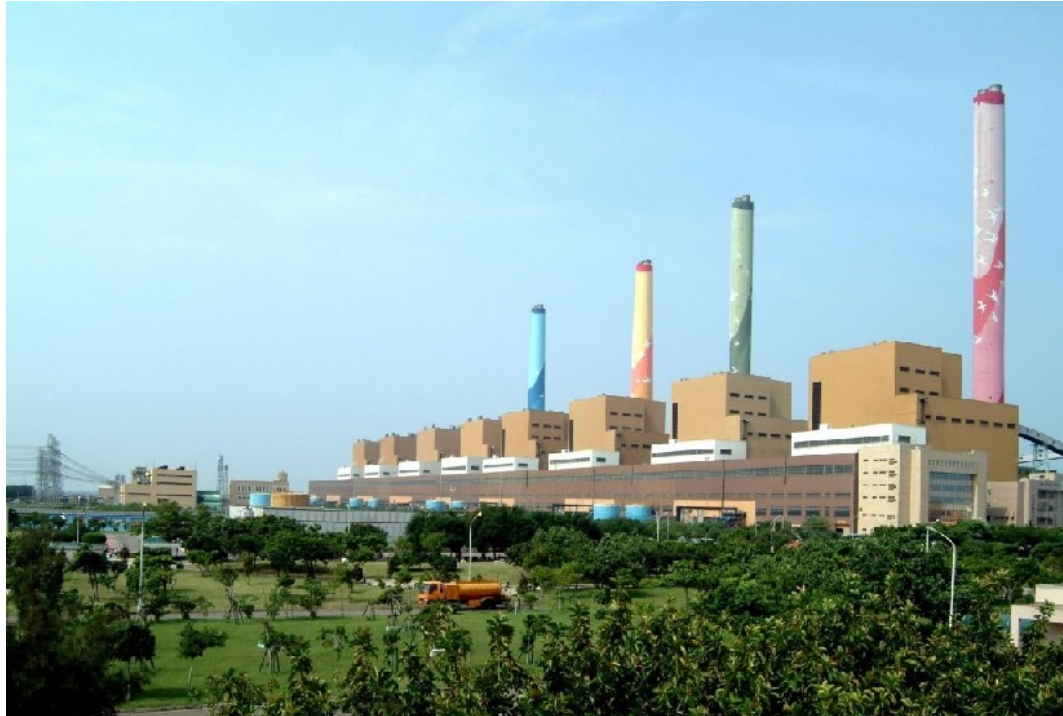
Figure 10 - Taichung coal-fired power plant (image from http://tpcteps.myweb.hinet.net/ )
