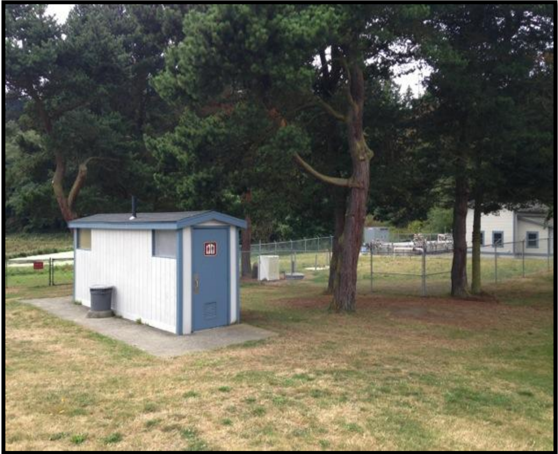
Figure 46. Fort Flagler State Park wastewater treatment enhancement project.
