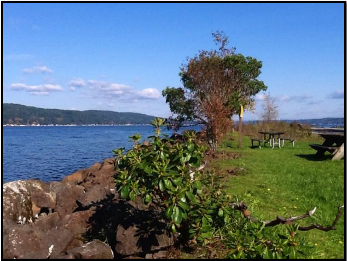
Figure 57. Twanoh State Park's armored shoreline scheduled for restoration.
