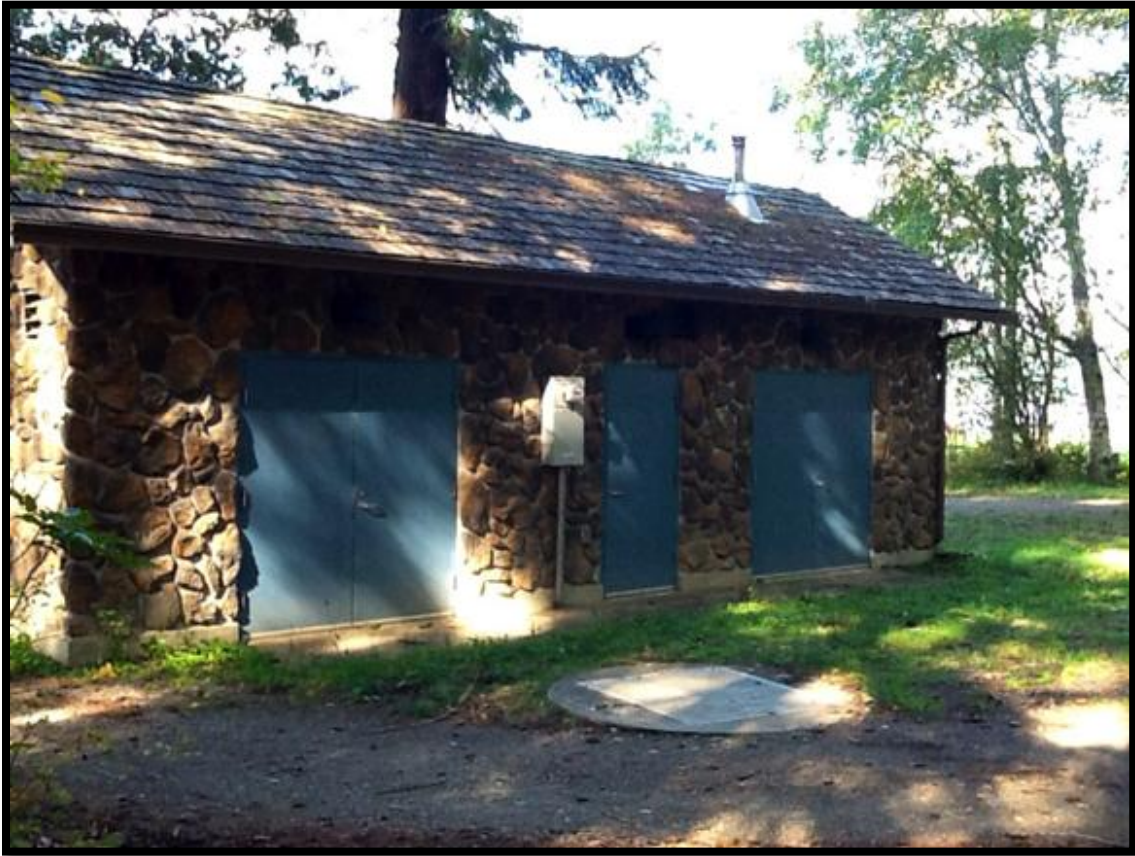
Figure 55. Twanoh State Park new wastewater treatment facility on site.
