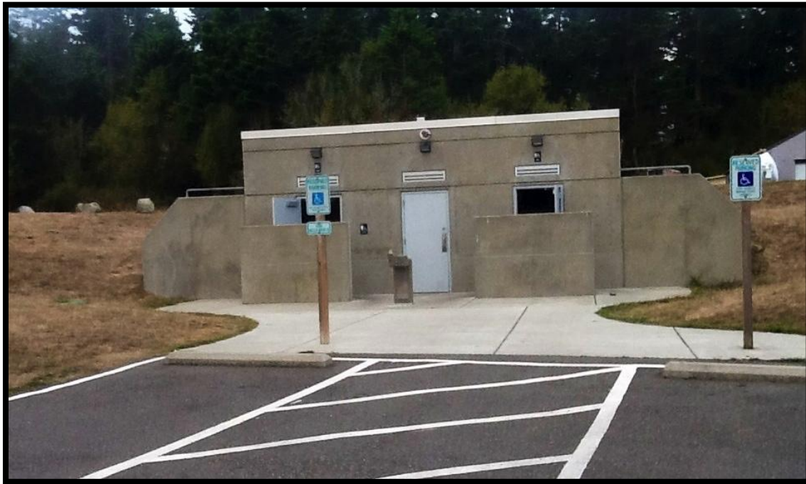
Figure 84. Fort Casey State Park's new restroom facility in lower part of park.
