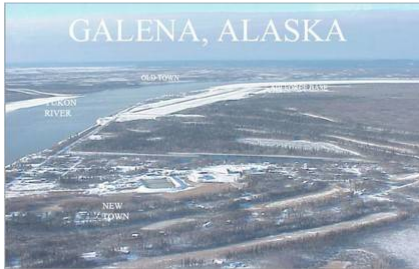
Figure 4.1: Aerial view of Galena, Alaska. 237
