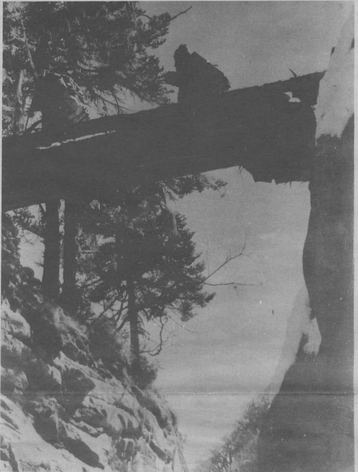
PORTERS CROSSING Imya Khola two days from Base Camp.
