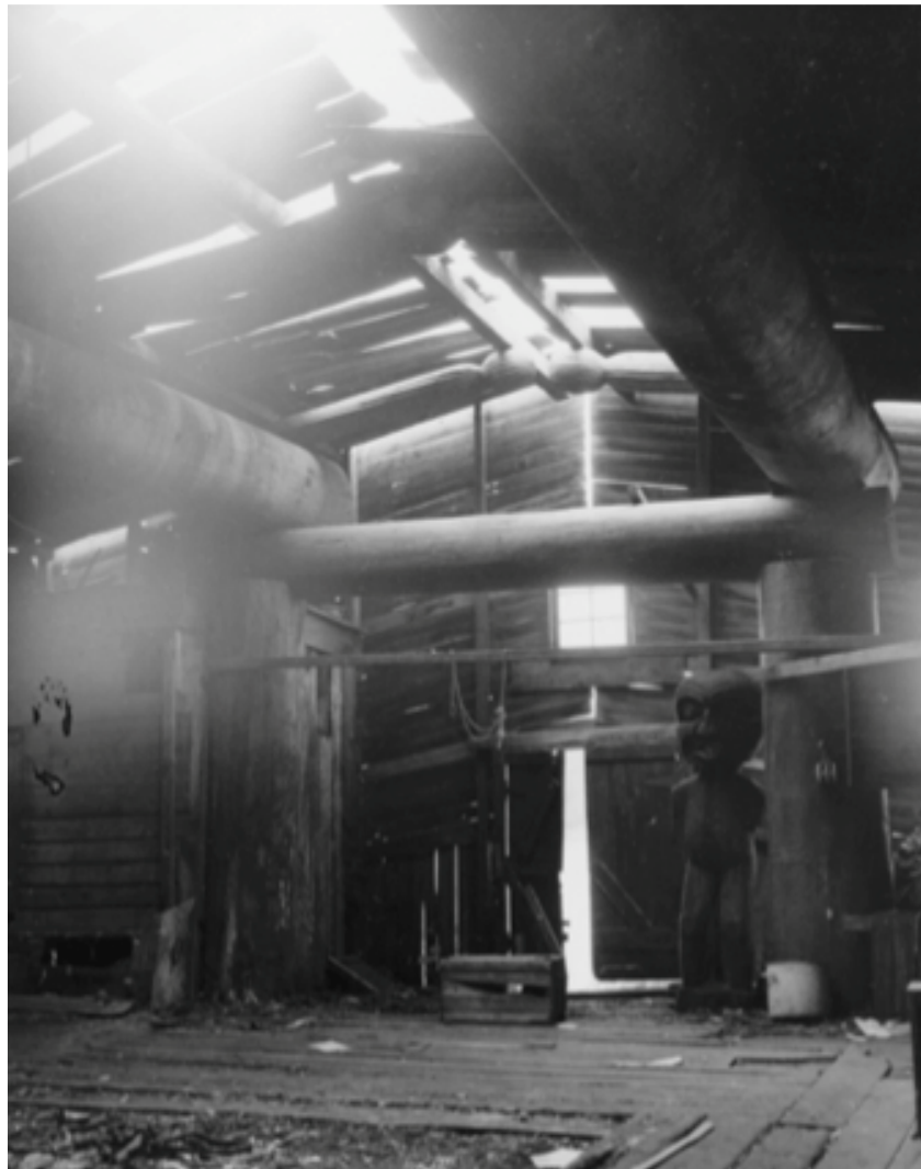
Interior of Kwakwaka'wakw four-beam longhouse, Blondin Harbor, British Columbia, 1951? National Museum of the American Indian.
