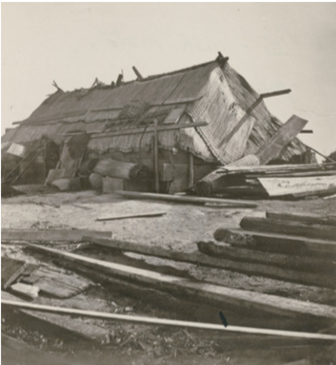
Esquimalt dwelling. Temporary shelter covered with woven mats for long-distance travel. Planks shown in foreground. Vancouver Island 1880. National Museum of the American Indian.
