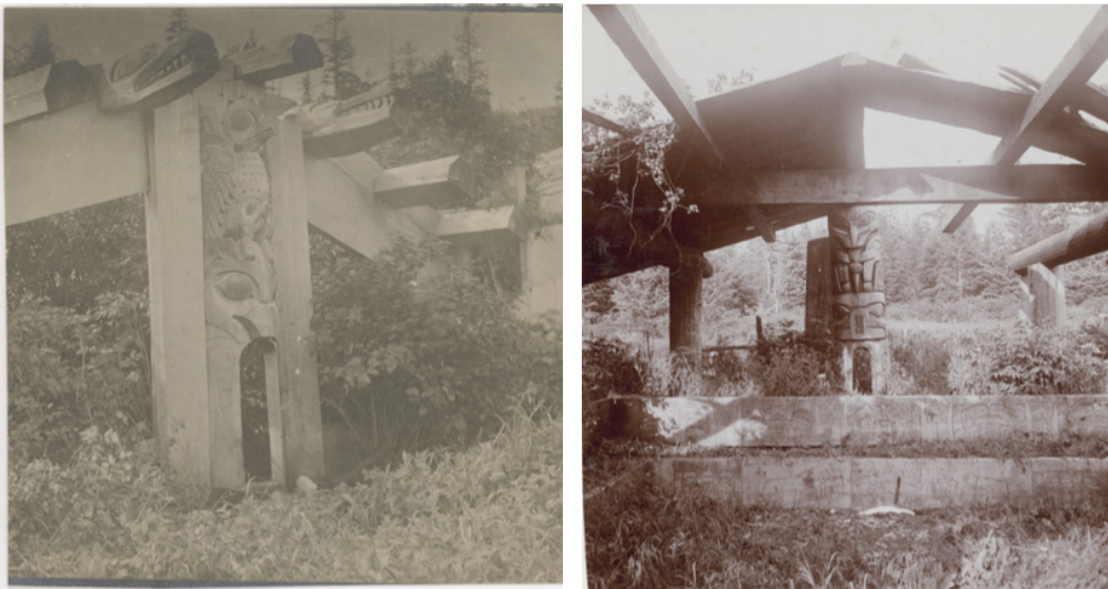
Photo on the left: Haida six-beam frame and entryway. Haida Gwaii 1897, National Museum of the American Indian Photo on the right: Tlingit four-beam frame, Prince of Whales Island. Date unknown NMAI
