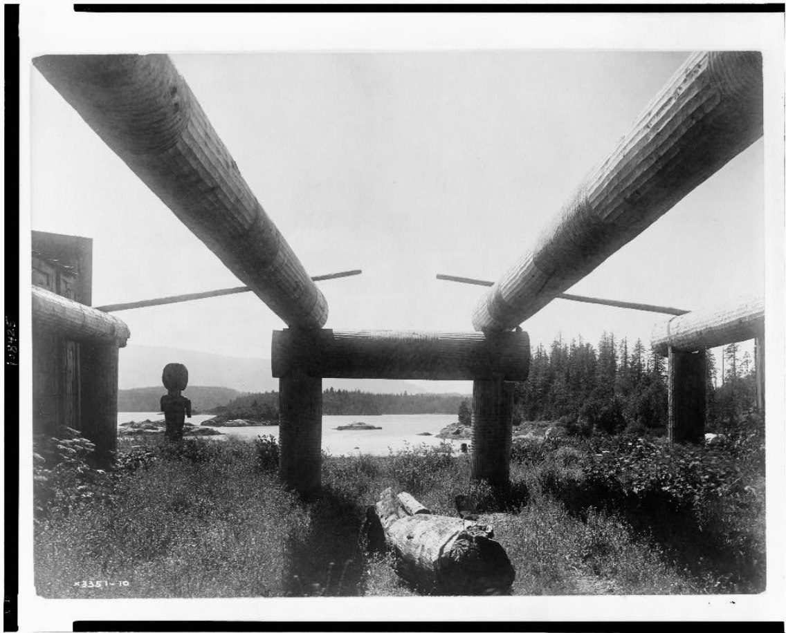
Kwakiutl 4-beam house frame 1910, Library of Congress Note: Notice the adze marks on the rafters, this was done to “even out” the beams making them essentially the same diameter from end to end. This shows the gable frame style of house, essentially two shed-roof houses
