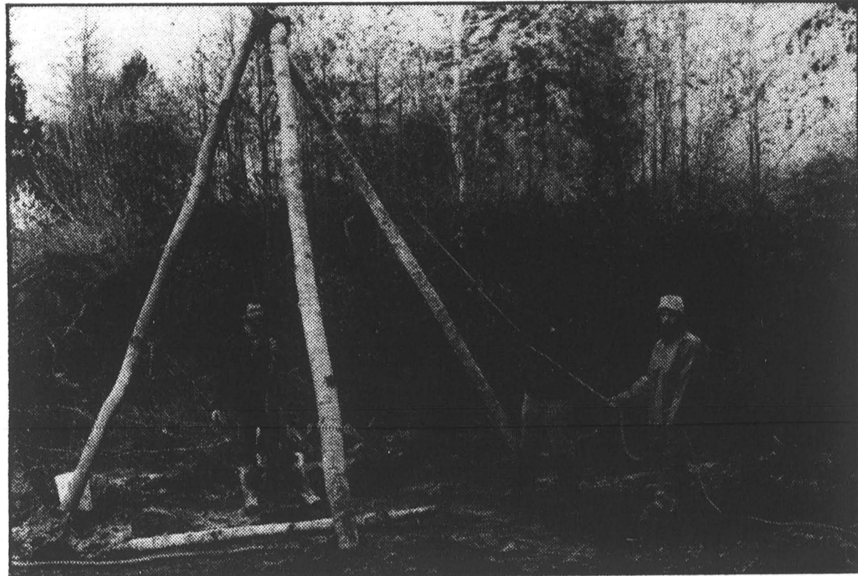
Cliff Missen, Gabriel Saytoneh, and an unidentified assistant demonstrate tripod technique of well drillings.
