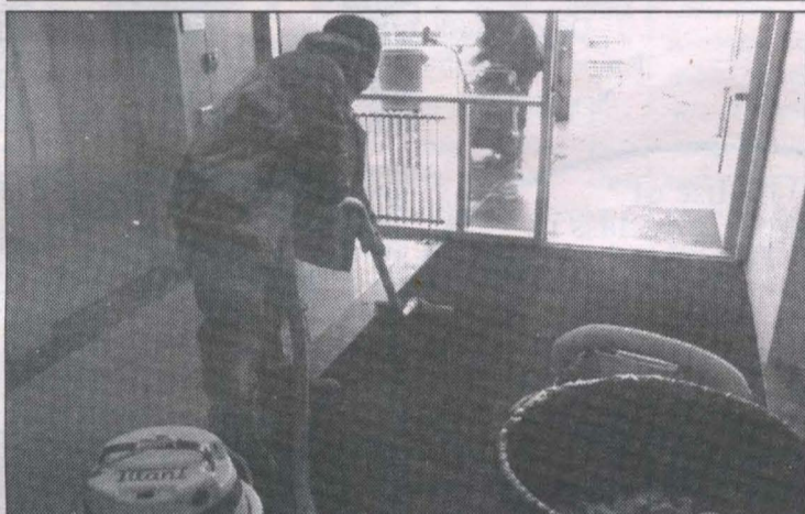
CUSTODIANS CLEANED UP THREE INCHES OF WATER ON THE 3RD FLOOR OF C BUILDING. PHOTO BY BOBBY WILLIAMS
