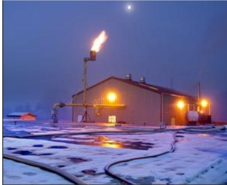
Figure 21. Qualco digester flaring excess methane (Bartley, 2012)
