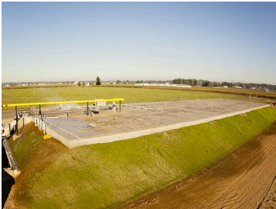
Figure 15. Edaleen Cow Power's plug-flow digester (Andgar, 2012b)
