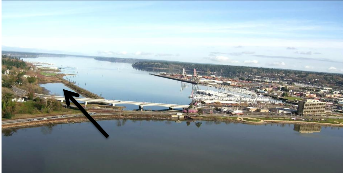
Figure 6.6 Divert sediment by installing a culvert and creating a channel to allow flow to enter basin behind railroad track. Allow the basin to fill and while this process is occurring, modify the dam's operations and the structure so that sediment can be deflected from the Port of Olympia. (Aerial Images NW)
