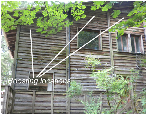
Figure 4. Roosting locations on south wall of Farmhouse on July 6, 18 & 22.
