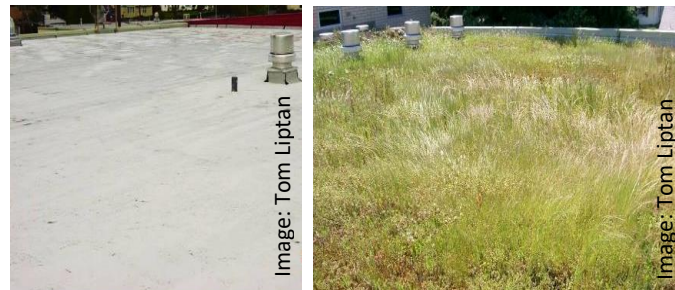
Figure 1. A cool roof next to an ecoroof in Portland, Oregon.
