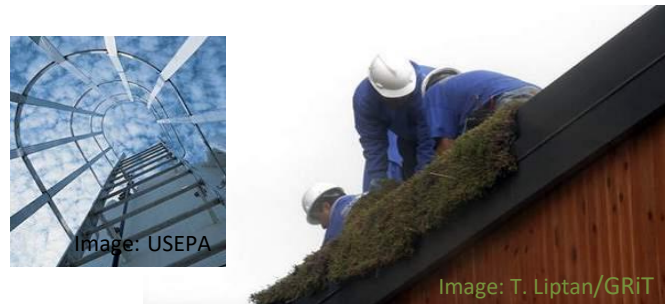
Figure 8. Safe access to green roofs presents limitations.
