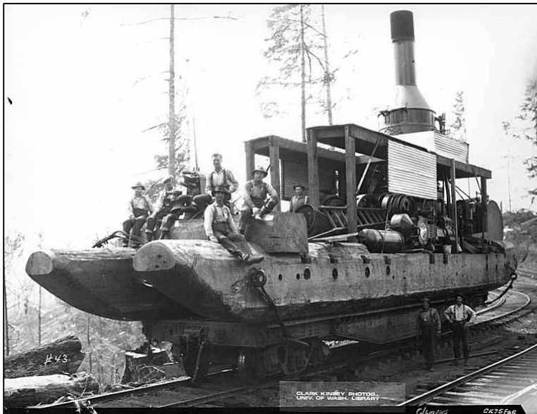
Figure 6. Example of a steam donkey. The timber of the West provided an ample supply of large skids such as the ones shown here. Photograph by Clark Kinsey (UWL, 2015).
