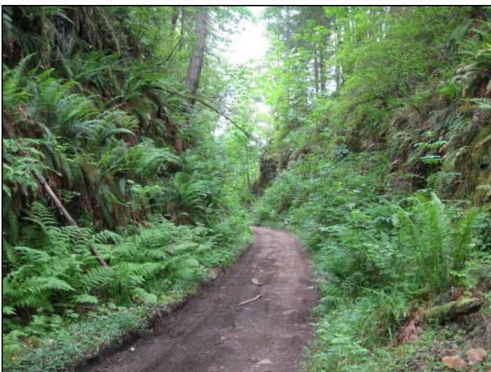
Figure 29. An extreme example for Capitol Forest, this through cut near Mud Bay Logging Company's Camp 2 is greater than 40 feet deep through solid rock. Photograph by Lee Stilson (Stilson, 2010A).
