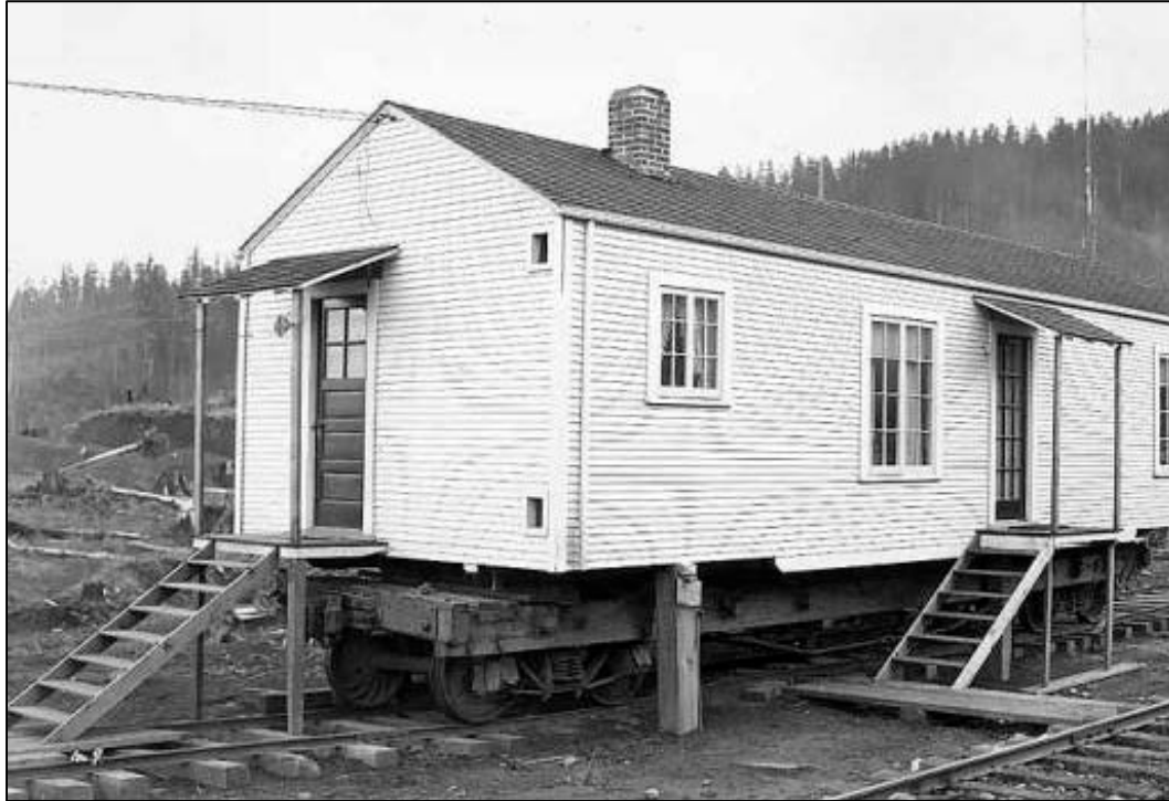
Figure 1. Example of a logging camp bunkhouse on a railcar. Having moveable structures allowed for quick movement of logging camps to new locations. Photograph by Clark Kinsey (UWL, 2015).
