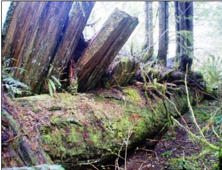
Figure 16. Portion of the Wedekind Dam. The dam was constructed from one large log with planks placed against the log to impound water and sediment (Ferguson, 2011D).
