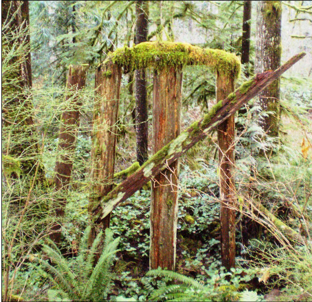
Figure 43. Looking south from end of grade at the standing portion of trestle remnants found in aggregate segment E3. Photograph by author.
