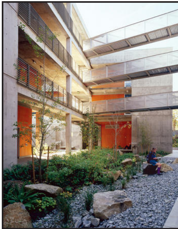
Photo 2.1 Seminar II Building at TESC. The Seminar II building earned LEED gold standard. This photo illustrates stormwater drainage that incorporates a themed teaching Garden, and outdoor hallways eliminating the need for additional lighting and temperature control. Photo credit: Lara Swimmer.
