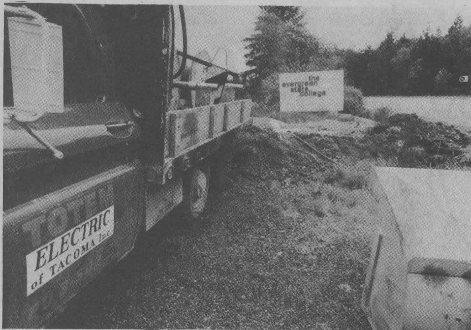
Light standards being installed on the Parkway
