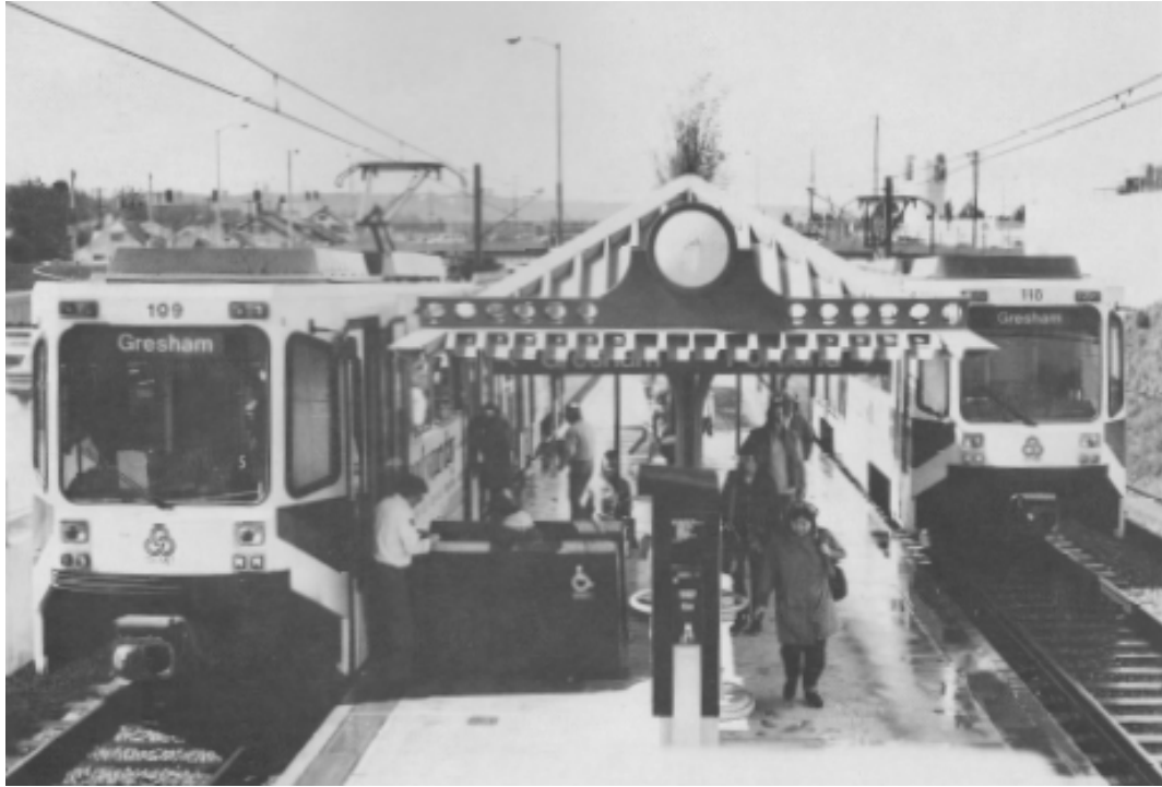
Figure 12: Two MAX trains at the Hollywood Station, November 1986 (Hare, 1989, p. 55)
