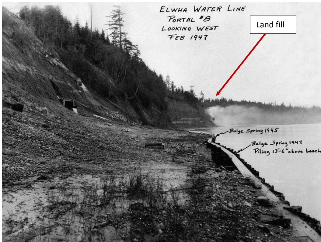
Figure 11. Looking west along the base of the Elwha bluffs towards the City of Port Angeles landfill in the distance, 1947. The photo shows a portal (center) for the industrial water line buried along the toe of the Elwha bluffs and protected by shoreline armoring (right). Photo courtesy of Coastal Watershed Institute.
