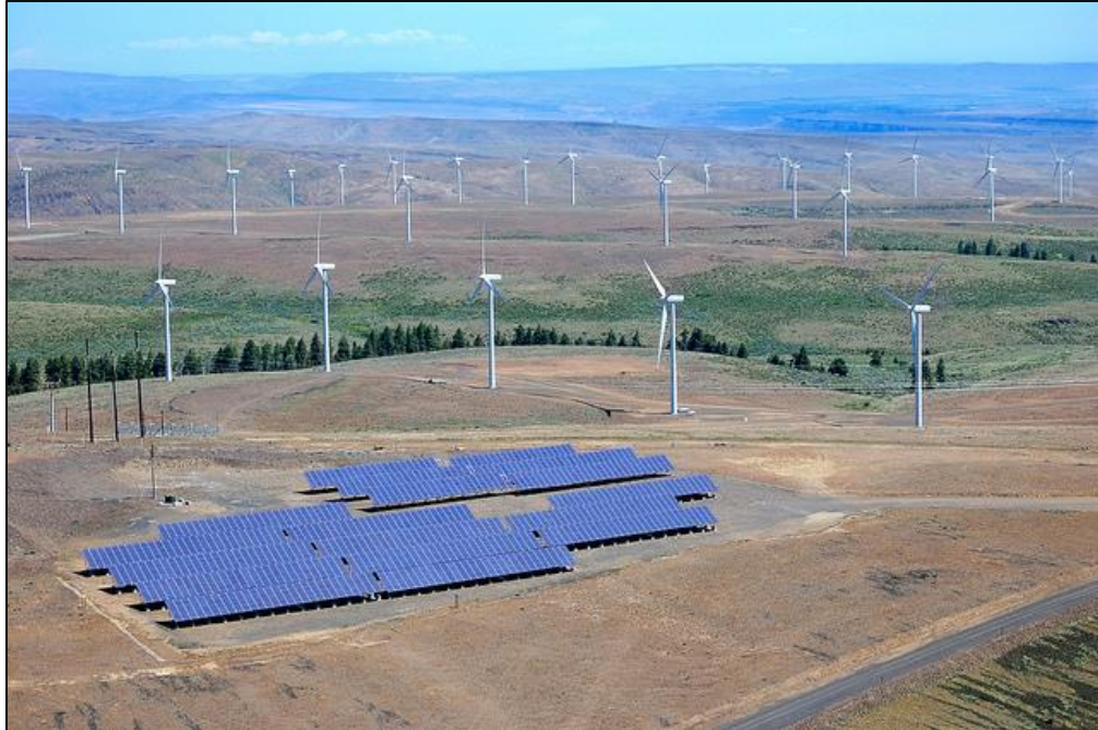
Figure 1. Wild Horse Wind and Solar Facilities (Ellensburg, WA)
