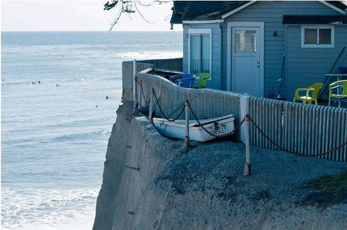
Figure 2. Seawall protecting private property along East Cliff Drive.
