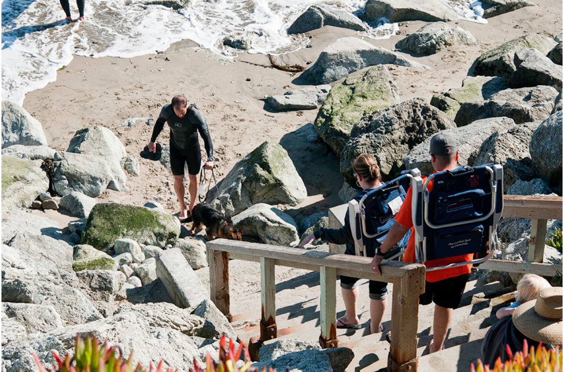
Figure 5. Dangerous public access point constructed as part of the Pleasure Point Seawall Project at 38 th Ave.
