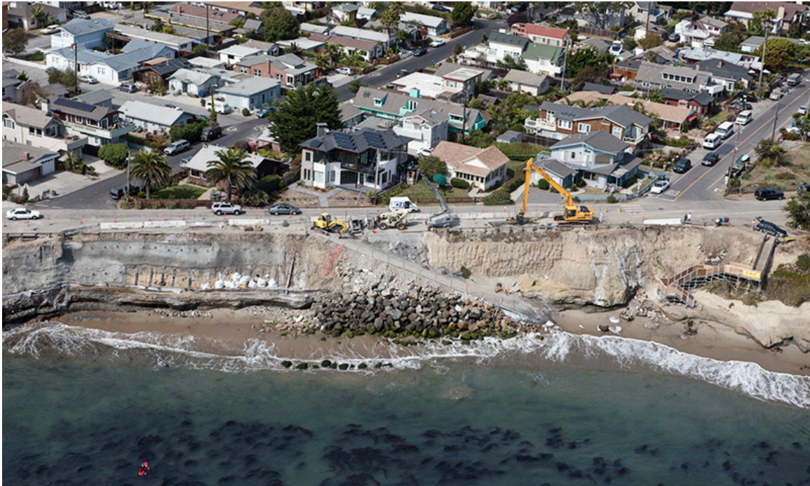
Figure 1. Pleasure Point Seawall construction at 38 th Ave. (California Coastal Records Project)
