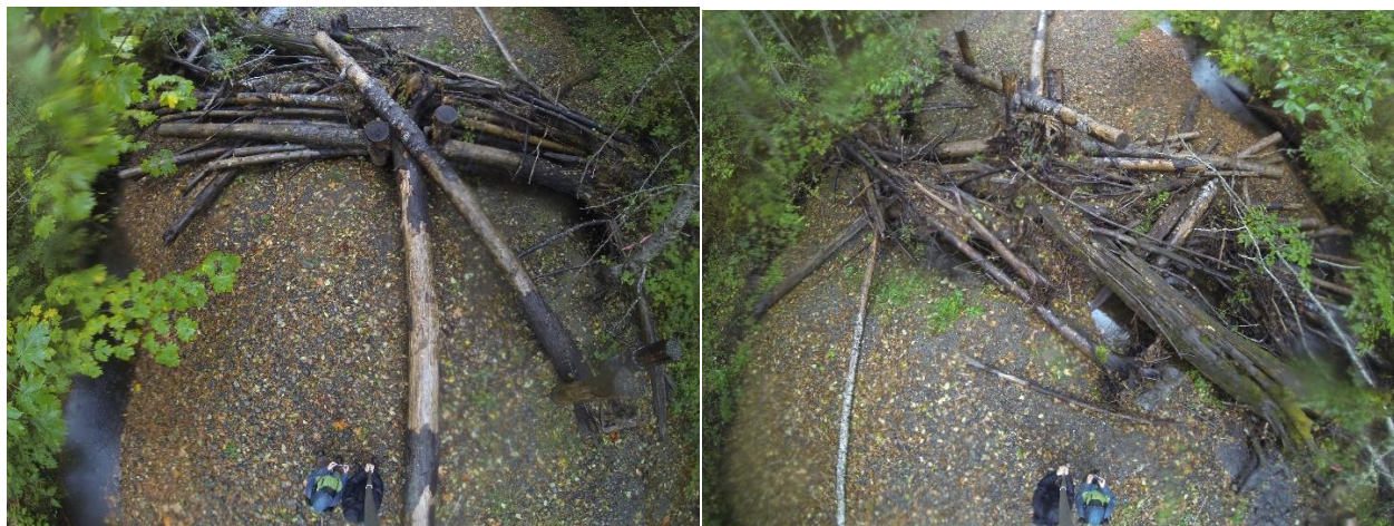
Figure 10. Example of wood structures built during phase 1 of the lower BBC restoration. This set of structures were built around posts driven into the streambed with a backhoe and included 'slash bundles' of smaller logs bound together with rope at their base (the complete restoration design may be viewed at PRISM 2018). Photographs are of the same structure depicted in the plan and were taken two years after construction in 2015 - facing upstream (left) and downstream (right). A backwater pool is present underneath the wood in the photographs and this structure has wracked additional wood since construction. Upper image (blue arrow indicates flow direction from McCullough 2015).
