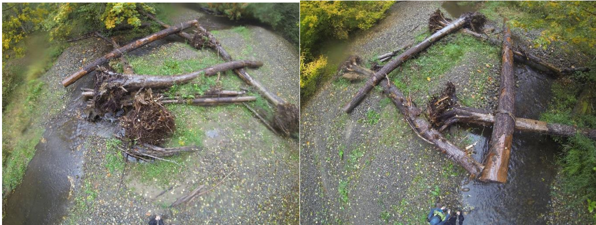
Figure 11. Example of wood structures built during phase 2 of the lower BBC restoration. This set of structures were placed by helicopter and included 'slash bundles' of smaller logs bound together with rope at their base (Seen best in center image on the left, the complete restoration design may be viewed at PRISM 2018). Photographs are of the same structure depicted in the plan and were taken one year after placement in 2016 - facing upstream (left) and downstream (right). The slash bundles associated with this structure is becoming buried in the sediment, a small pool is associated with the root wad in the middle of the left image, and aggradation of bed materials around the structure contributed to the activation of a previously abandoned channel reach (black arrow upper image). Upper image (blue arrow indicates flow direction from McCullough 2015).
