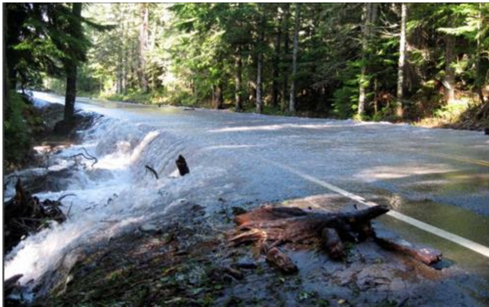
Figure 13. A new channel was formed on the Kautz Creek from the increased precipitation a mile upstream from the roadway (NPS, 2006)
