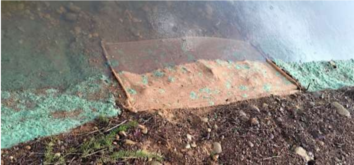
Figure 5.3 Plots 24 hours after seeding on March 10, 2016. Note migration of hydromulch, especially in plot at left. Hand broadcast sowing and hydromulching was performed on March 9, with hydromulch applied between 9:00am and 10:00am (seed was applied prior, the same morning). Low tide occurred at 1:11pm at 2.58 feet (MLLW), and the next high tide occurred 6:22pm at 14.35 feet.
