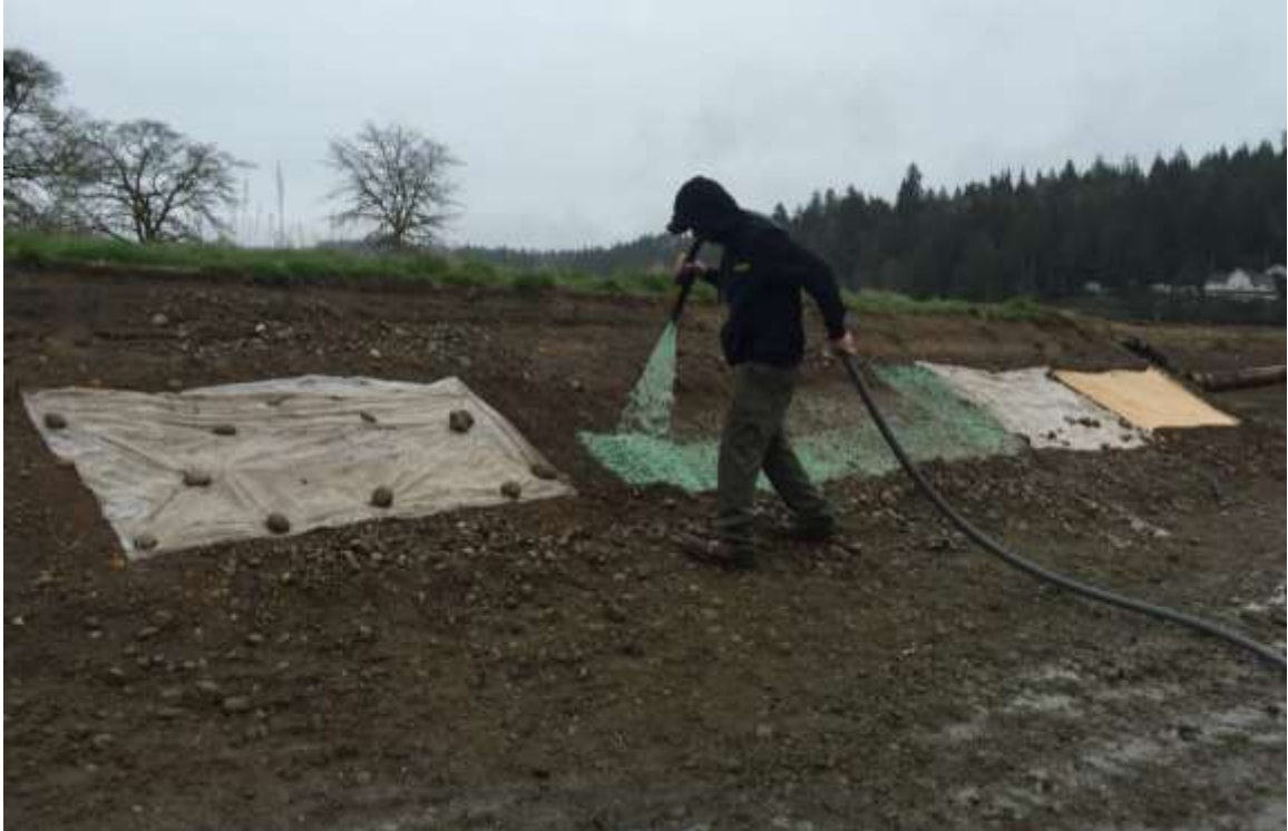
Figure 5.1 Hydromulching in progress on March 9, 2016.
