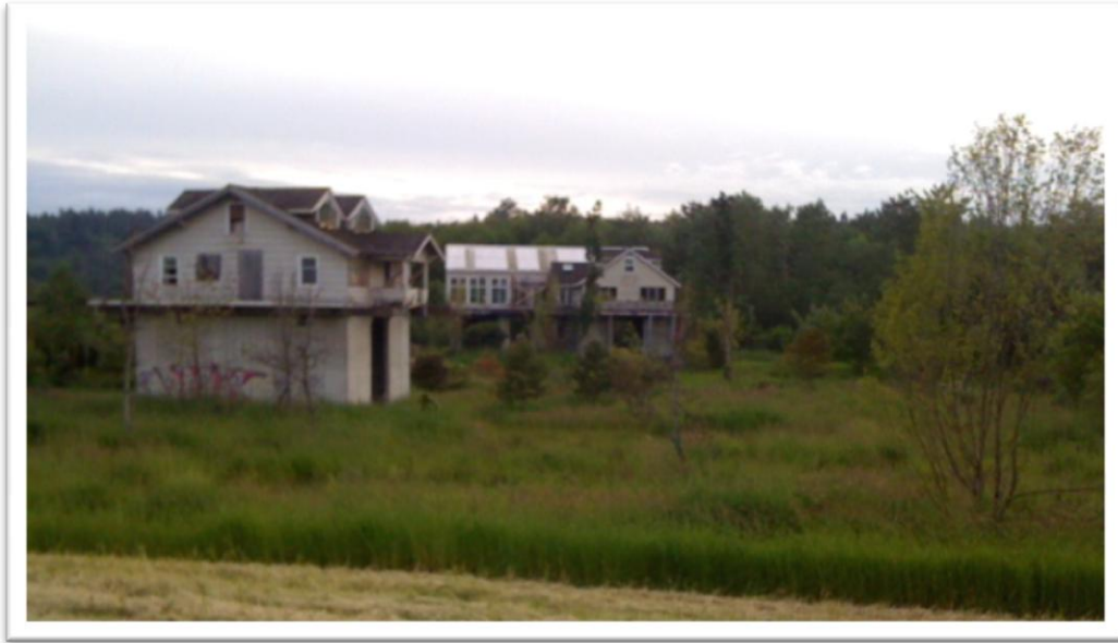
Figure 12. Snohomish homes built on stilts for flood disaster adaptation. Photo by Zoltan Grossman.
