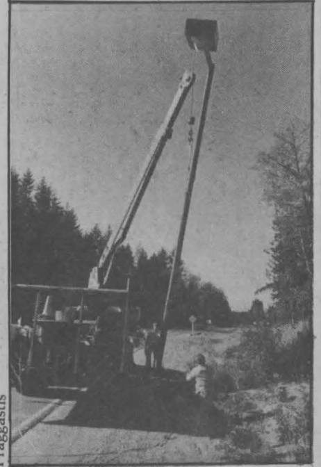
A crane erects one of the controversial parkway lights.
