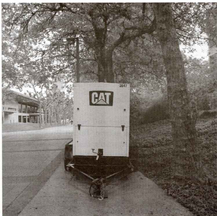
CAT generator being used in Lab II renovation. JASMINE KOZAK-GILROY
