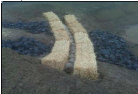
Bio-filter construction
