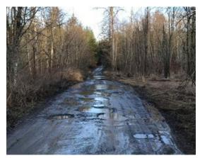
Figure 15: Degraded easement from increased traffic.
