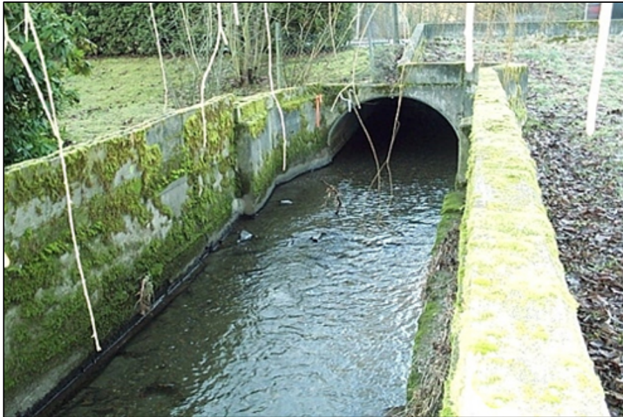
Figure 1: Shows a pre-project photograph of the South Fork of Thornton Creek flowing through a culvert underneath 35 th Ave. N.E. in Seattle, WA. Photograph provides an excellent example of channel armoring and the absence of floodplain connectivity. Source: Seattle Public Utilities ( http://www.seattle.gov/util/EnvironmentConservation/Projects/MeadowbrookThornton/Details/index.htm )
