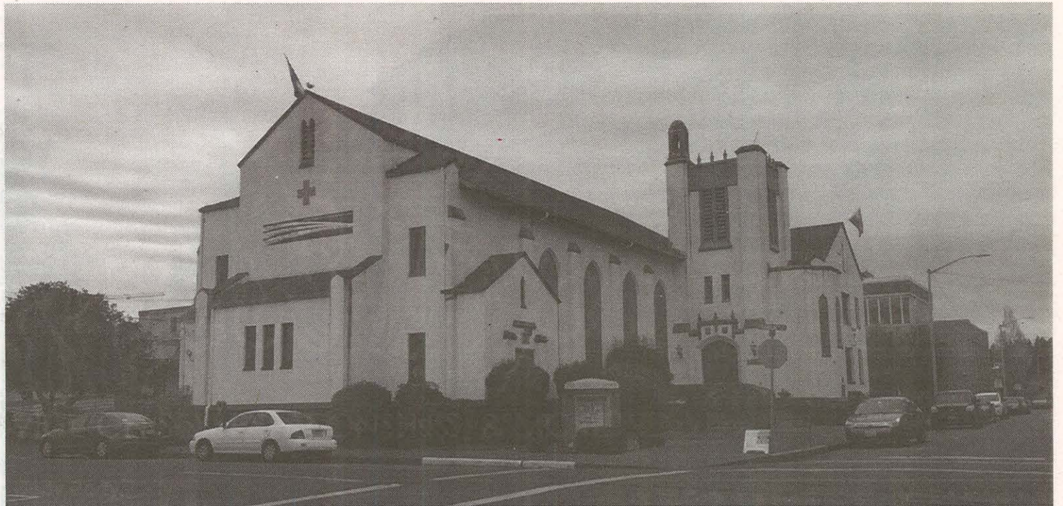
The shelter at First Christian Church was expanded into an emergency storm shelter by volunteers. JON FITZGERALD.
