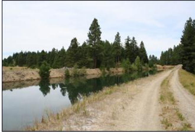
Figure 11: A road running alongside the KRD Main Canal providing easy access for maintenance and installation
