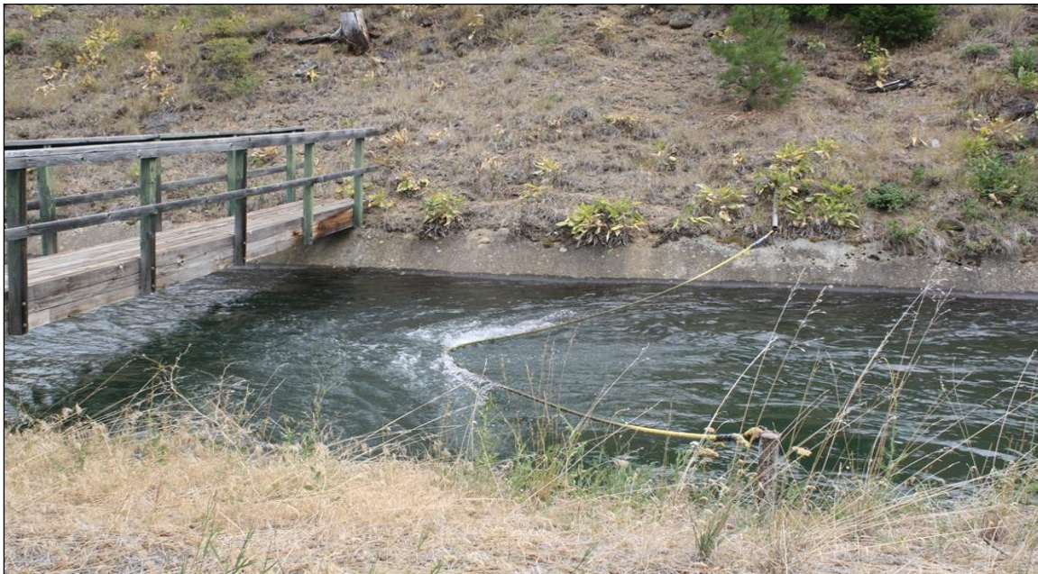
Figure 19: Site C of the KRD North Branch Canal
