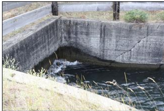
Figure 10: A siphon in the KRD Main Canal
