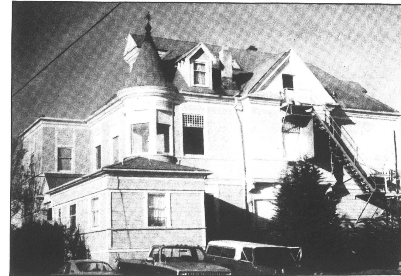
The Uptown Apartments, home to many students, may be the next to go.
