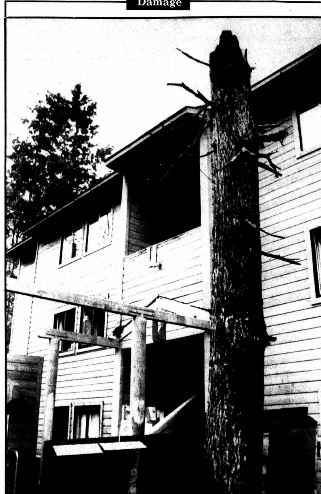
U-dorm's entryway was damaged by a tree during the storm on Jan. 20. photo by Seth "Skippy" Long.
