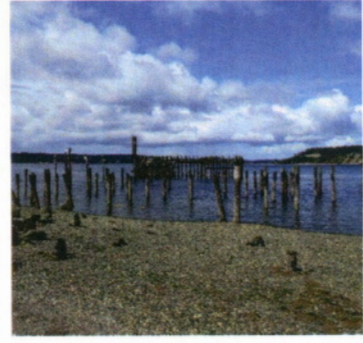
8c. Pilings from an abandoned ferry terminal, in the nearshore habitat of the armored section of Titlow Park
