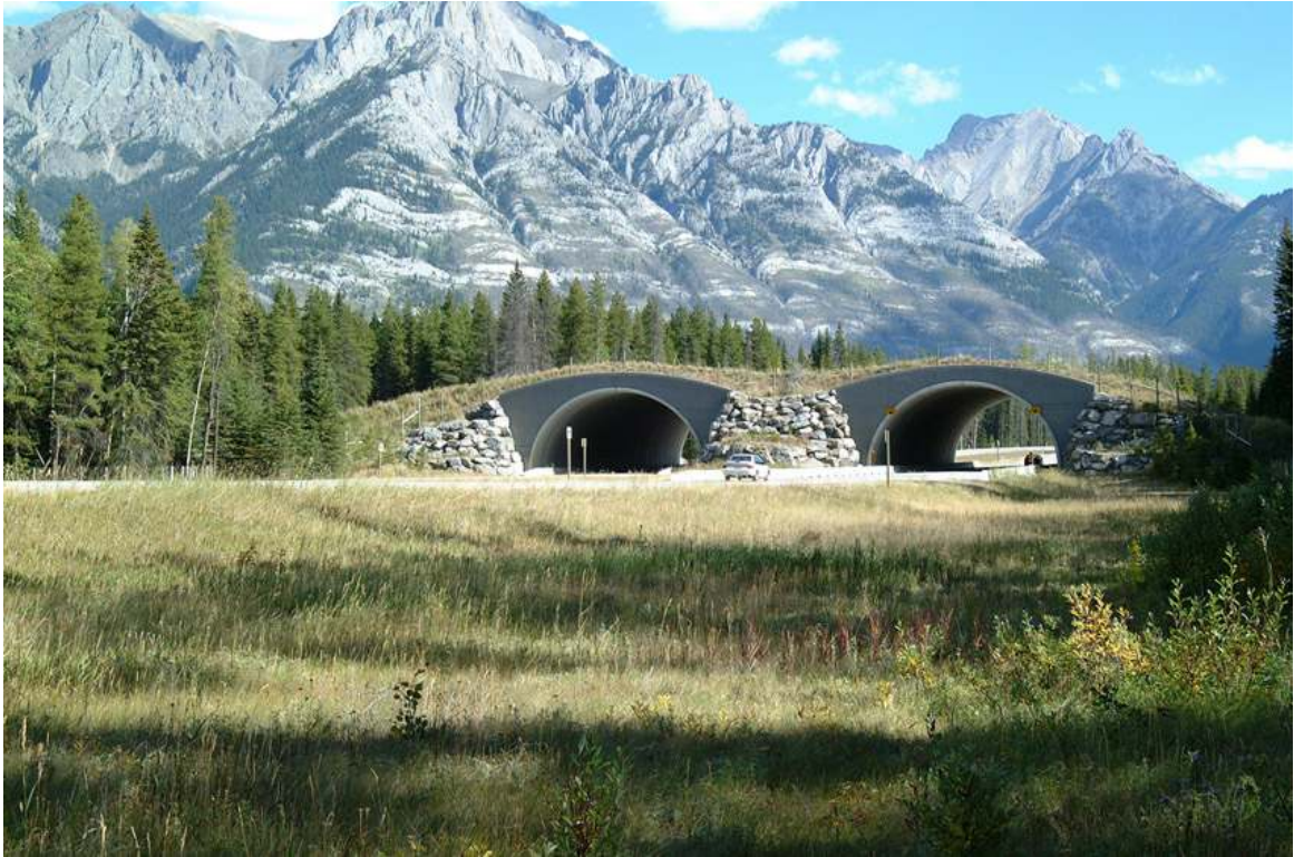
Figure 4. An animal crossing overpass structure in Banff National Park (ARC solutions.org, 2012)
