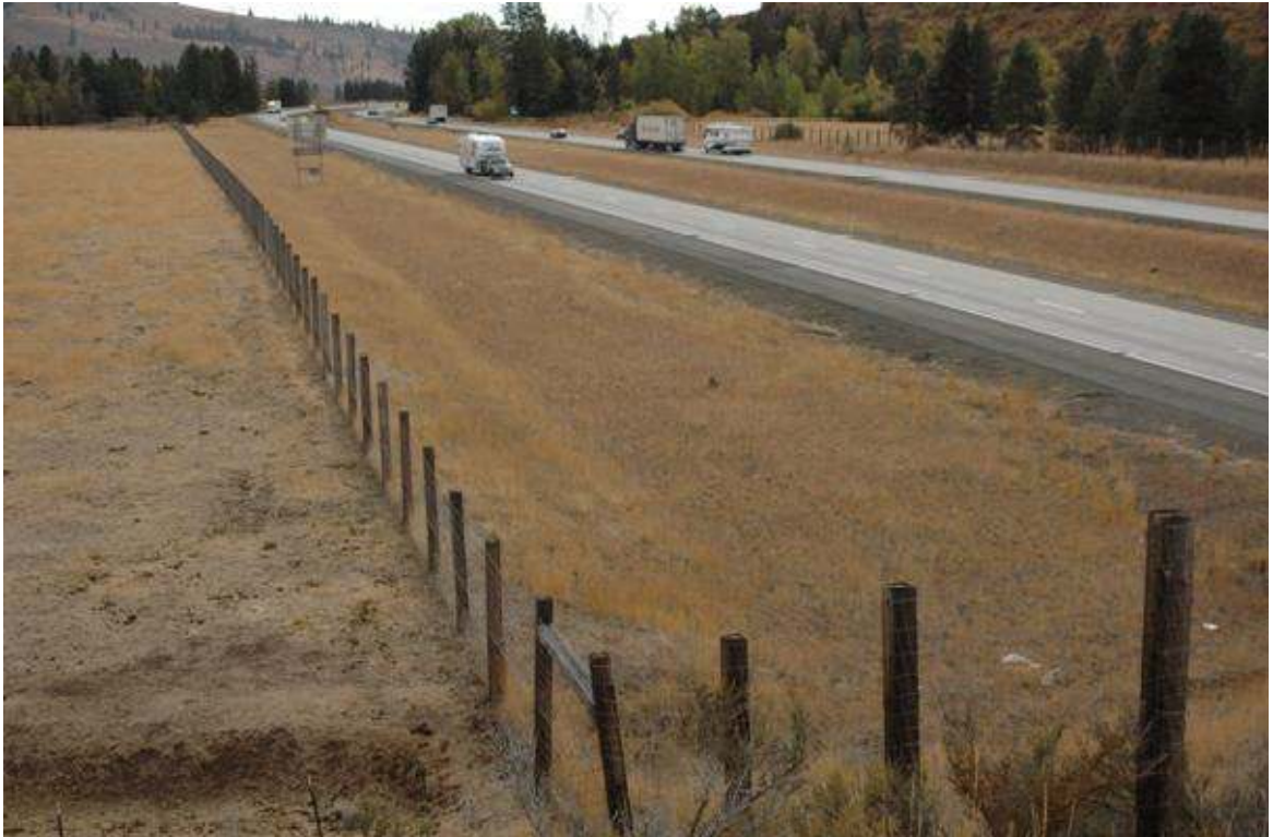
Figure 2. Wildlife fencing installed to keep deer and elk off of the roadway ( www.wsdot.wa.gov , 2012.)
