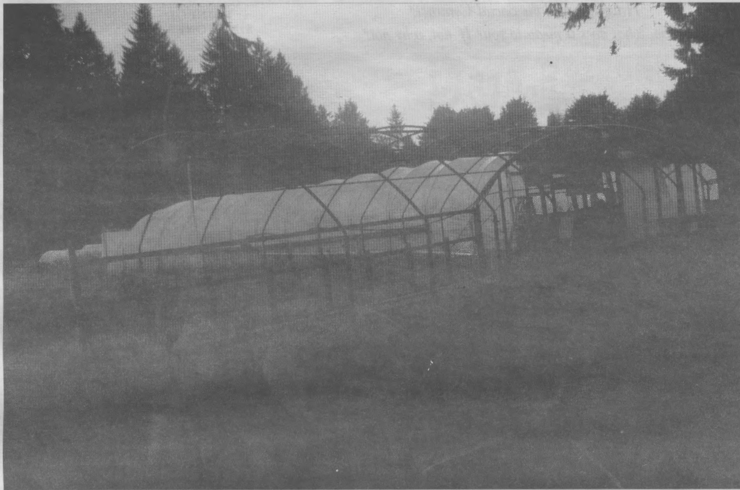
REMNANTS OF THE HEATED GREENHOUSE AFTER A RECENT FIRE
