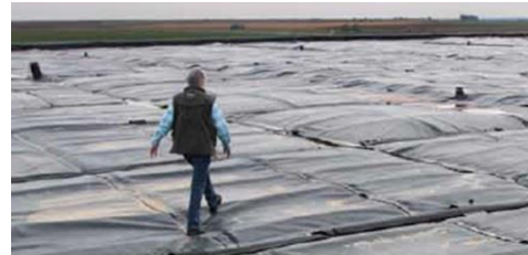
Figure 17: J.R. Simplot Digester (Source: J.R. Simplot)
