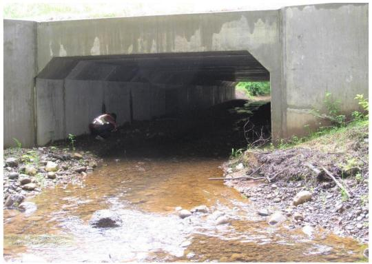
*Note*. This image depicts a type of medium wildlife bench known as a stream simulation structure, a type of crossing structure that allows both animals and a creek or river to pass underneath a roadway as if they are passing under a bridge. Source: WSDOT, https://wsdot.wa.gov/sites/default/files/2022-09/Wildlife-FishPassage-HabitatConnectivityReference.pdf
