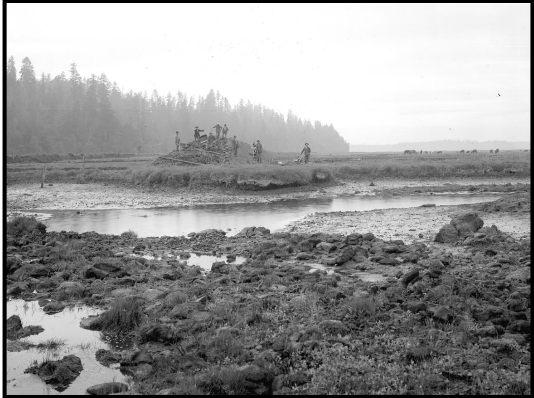
Figure 3: Nisqually Dike Construction (Source: WA State Historical Society)
