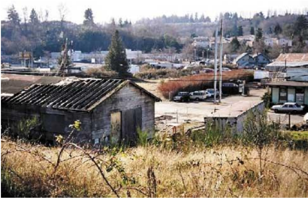
Figure 3: The brownfield site before the redevelopment process at Rainier Court. Hazardous chemicals from illegal trash dumping contaminated the site. (Retrieved from: http://www.geoengineers.com/project/rainier-court-brownfield-development )
