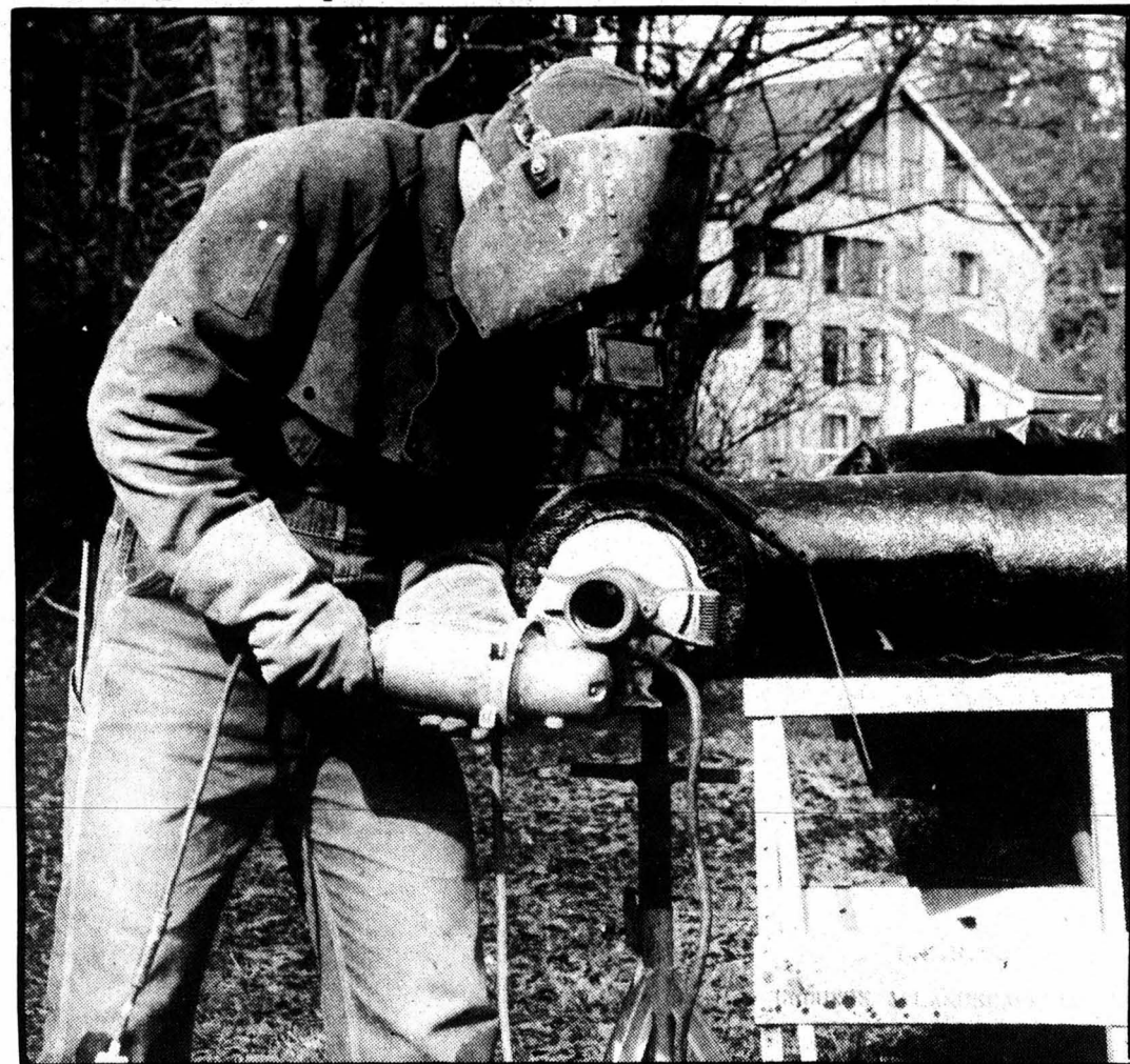
As the piping proceeds the pit progresses. photo by David Mattingly
