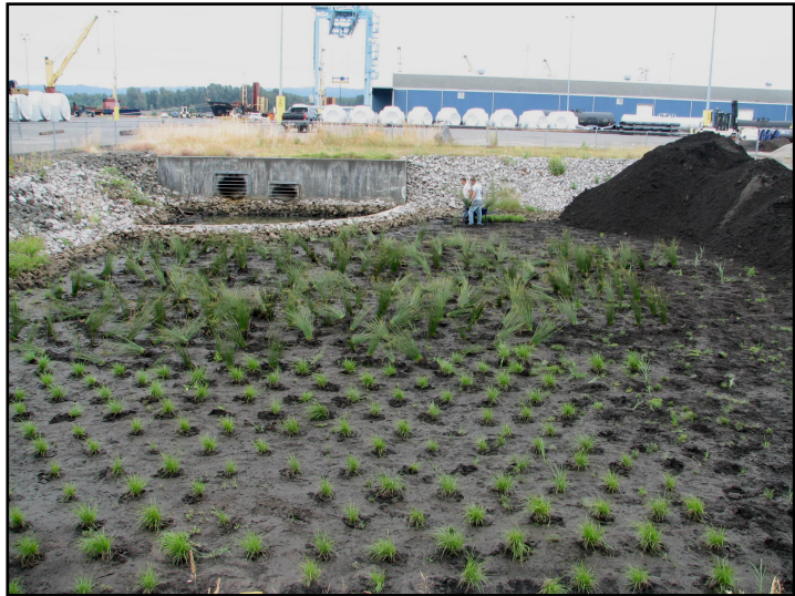
Figure 2: Bioretention facilities are engineered LID features that reduce stormwater flow and provide water treatment.
