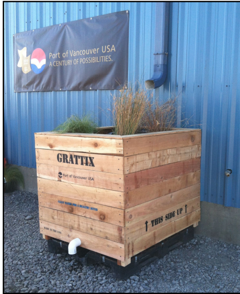
Figure 6: The innovative Grattix invented by PV employees removes 90-95% of zinc from roof runoff and is simple and inexpensive to build and maintain.
