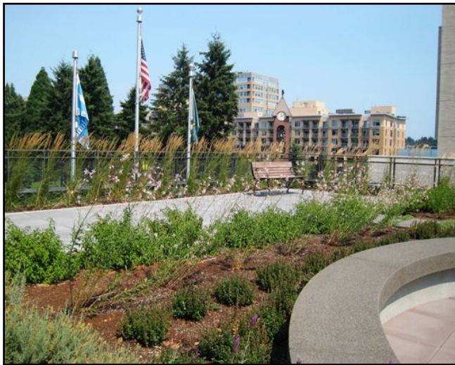
Figure 3: Green roofs provide stormwater abatement for rooftop runoff. Some green roofs provide outdoor living space.
